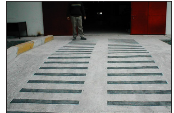
Finished ramp surface
